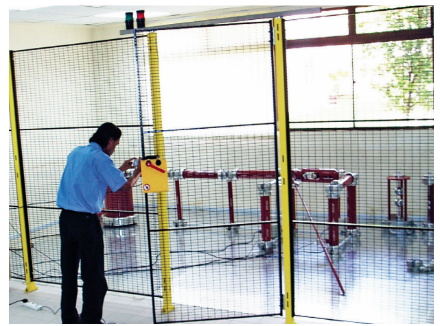
Installation of Safety Fence
